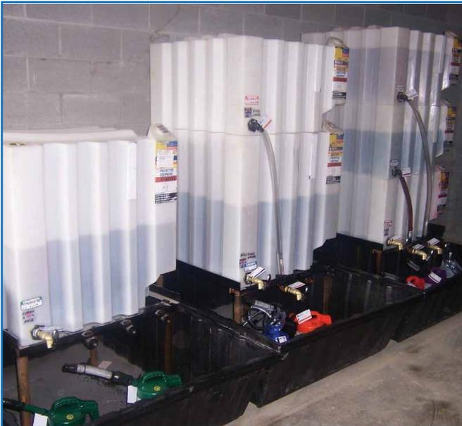
Tote-A-Lube storage tanks and Oil Safe transfer containers keep lubricants clean and contaminant-free
